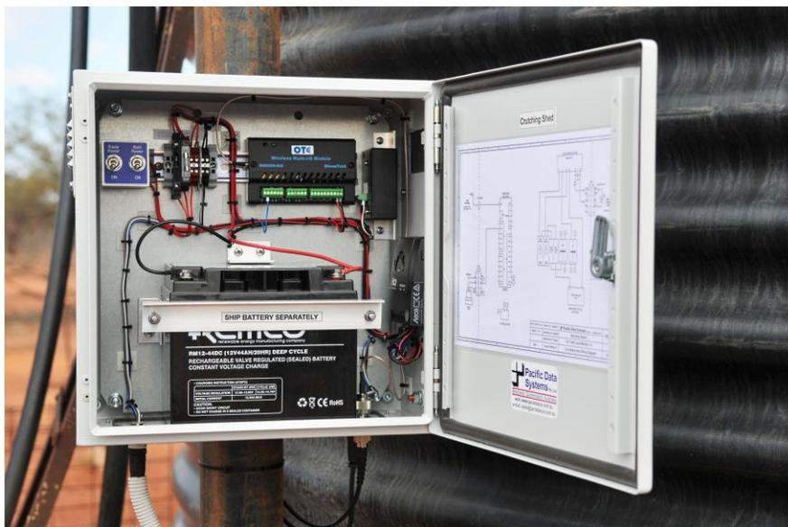
The simplest method of collecting field data is using a wireless point-to-point system that provides either uni-directional or bi-directional I/O communication. Think of it as a system that replicates hardwired signals from point A to point B with zero software programming. This type of system works well when scalability is a non-factor and also when the operator prefers or only has the option of using raw signals to tie into a SCADA system.
