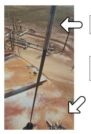
OleumTech's patented Resistive Sensor shown during inspection: no scale buildup.
