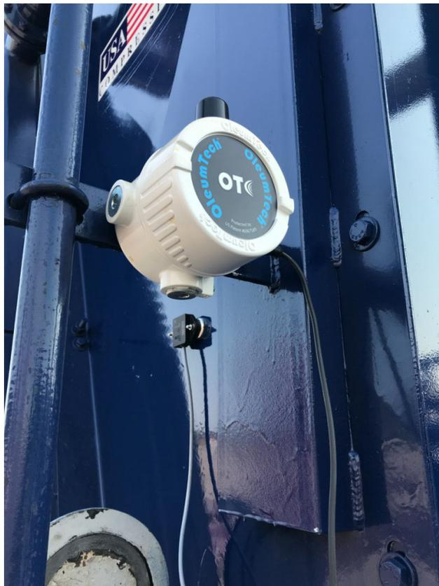
*Pictured: SM-JP4 V Wireless Vibration Transmitter installed on a compressor*
