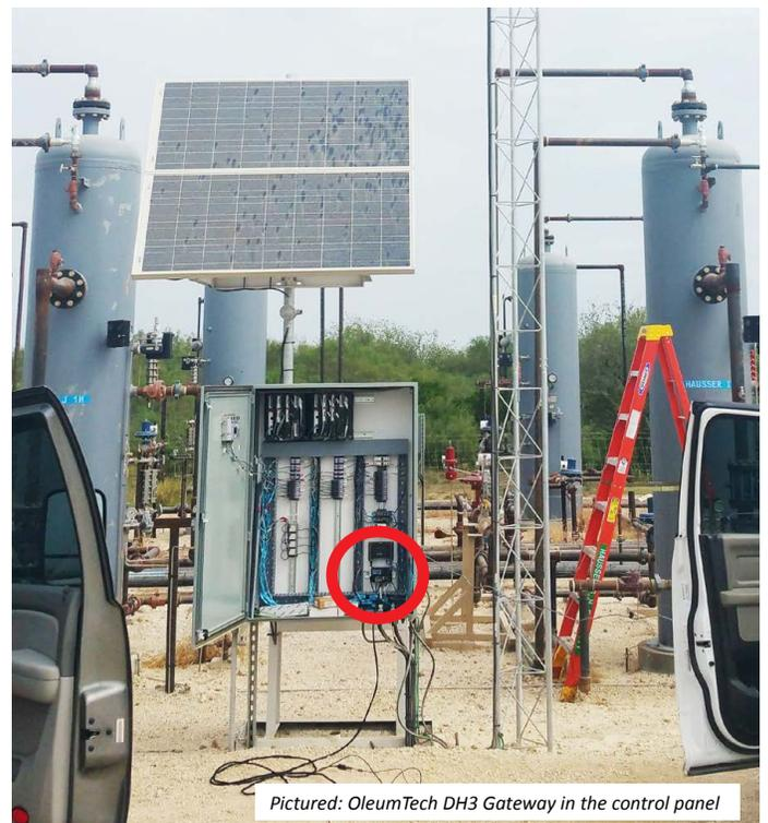
*Pictured: OleumTech DH3 Gateway in the control panel*
